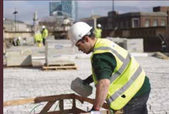
Above: 135,000 Granite setts/cobbles were imported from China. Knight Build had to organise the work to take into account the 10 week journey by sea. Knight Build kept the same personnel on all paving works, which were phased - this ensured a consistent, high quality finish.
