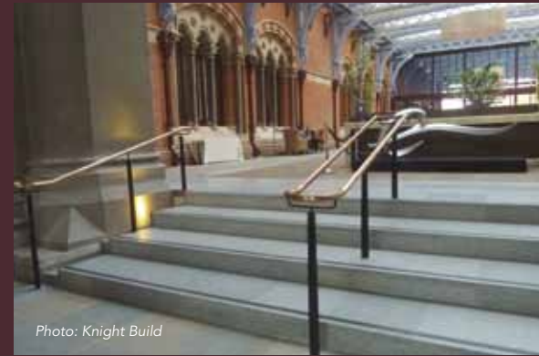
Below: Steps to the main Hotel lobby and reception and external forecourt York stone paving.
