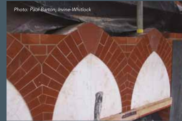
Above (both): Arches were built over polystyrene forms and these were re-used.
