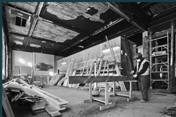
Left: The heritage floorboards – up to 6m in length – were de-nailed and planed on site, before being replaced. This task took six months!
