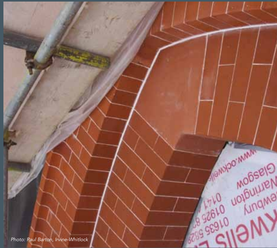
Above & left: On the Gothic arches, the joints are only 2mm wide and for these, a sand-free lime putty was used.
