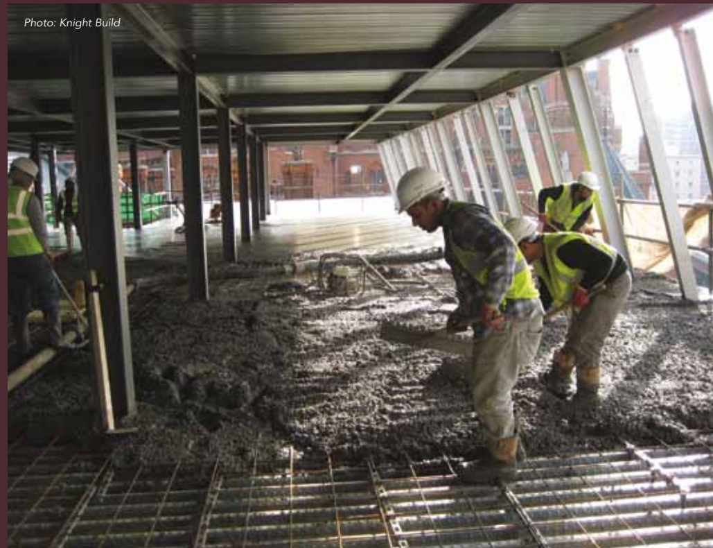
Left: Construction of reinforced concrete floors in the West Wing.
