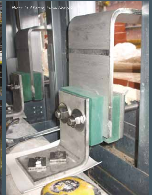
Above: Acoustic separation pads had to be designed and installed between the main steel frame and the brickwork ties.
