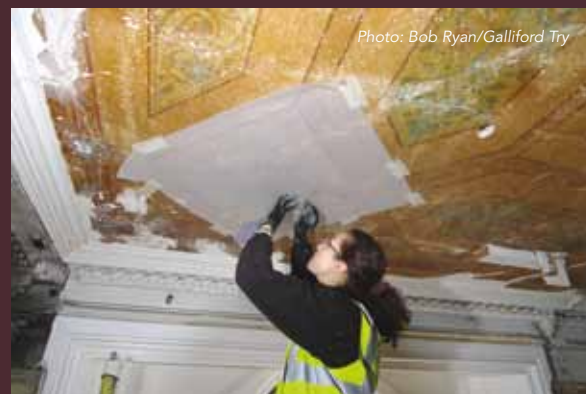
Far Right: Paints are hand mixed to match all the colours in the scheme and painted on numbered cards for easy reference and to avoid confusion. In the Ladies' Smoking Room scheme, 30 different colours were identified.
