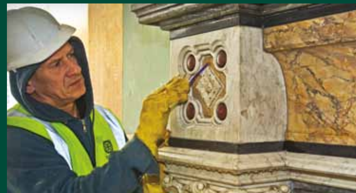
Middle: Fireplace before restoration. They all had to be removed to allow services, extractor fans and flues to be installed in the chimneys.
