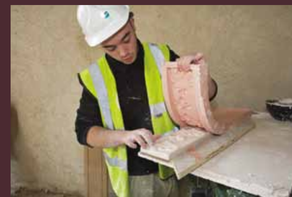
Below: Revealing the finished heritage plasterwork - moulds were made to enable accurate replication.
