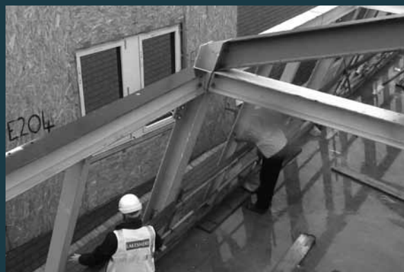
Below: Lakesmere installed one wall panel every thirty minutes – around six times faster than traditional methods of insulated wall construction.
