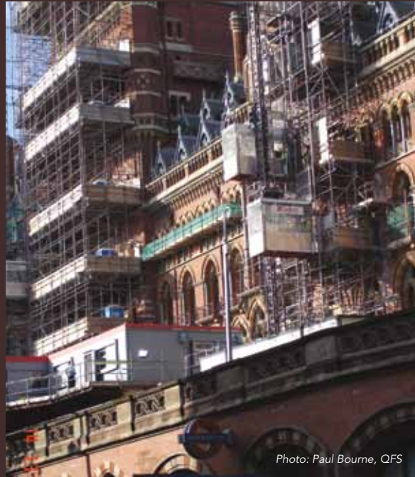
Below: Hoist arrangements and scaffold around the Penthouse on the Euston Road elevations.
