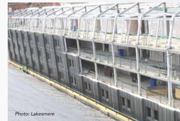
Above: Lakesmere's off-site manufacturing capability meant that significant costs were saved on scaffolding for the cladding.
