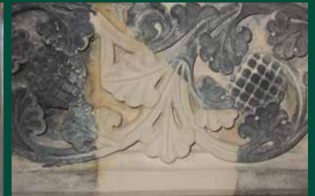
Above: Detail of stonework showing cleaned area. Trials and samples were essential to see what would work.
