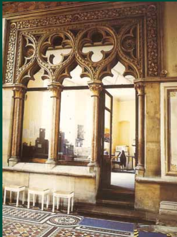
Above: With nothing but this postcard-sized picture as a guide, PAYE staff had to lay out the remaining pieces of the burnt screen and then recreate it in AutoCAD (detail below).
