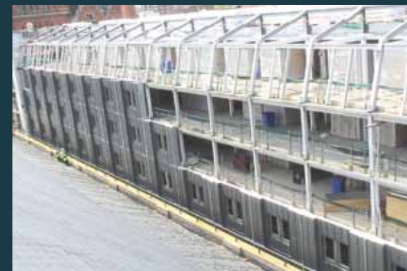
Right & far right: Lakesmere installed a total of 126 modular panels, covering 1,800m 2 of facade. The whole cladding operation was carried out in the time it would normally take just to erect scaffolding.
