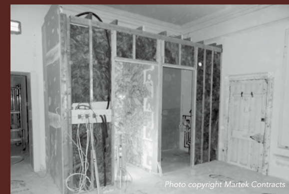
Above & right: Room pods – 'rooms within rooms' – during construction and completed. Note that the false walls are not attached to the ceiling. In the example on the right, the bathroom is situated behind the partition that forms the headboard for the bed.
