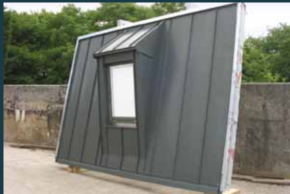
Left: The panels were pre-fitted with fixing brackets and windows and factory clad in sustainable, natural zinc to sympathetically blend with the original building.
